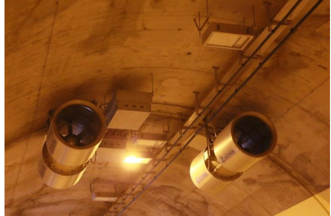
Figure 4. Structures under the ceiling in the Polana tunnel.
